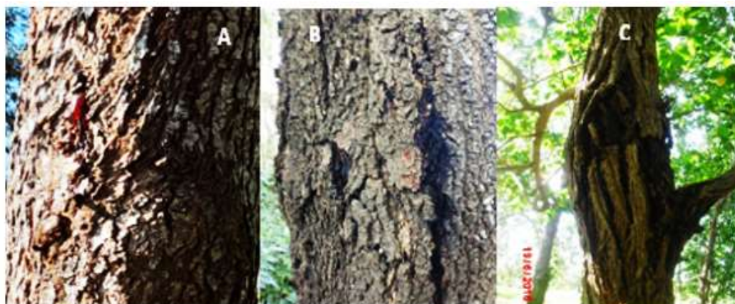
Figure 2. - Gummosis and bark cracking in Grevillea robusta (A), Gummosis and bark cracking in Acacia mangium (B) and Gangrene in Hibiscus elatus (C)
